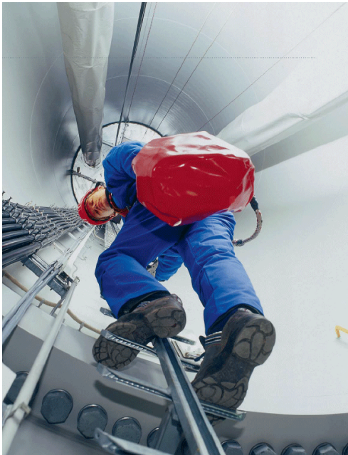
Figure 4: The insulated copper cables running down from the generator carry huge currents. (Courtesy of Enercon.)
